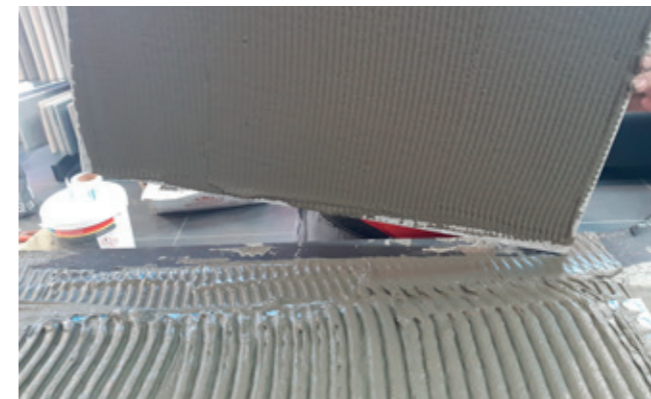
Fig. 10 – Buttering-floating bonding
