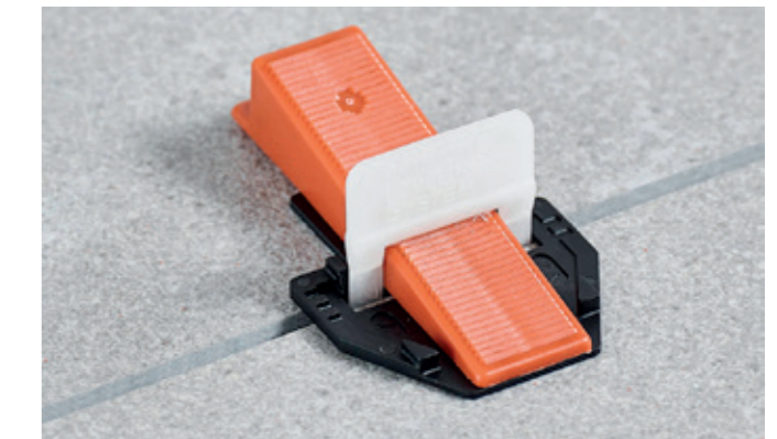
Fig. 11 – Washers under the levelling wedges
