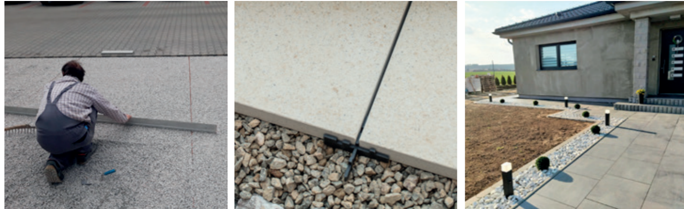
Fig. 28, 29, and 30 – Laying into gravel
